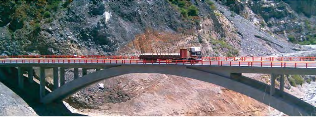
Puente Billinghamurst. Billinghurst bridge.
